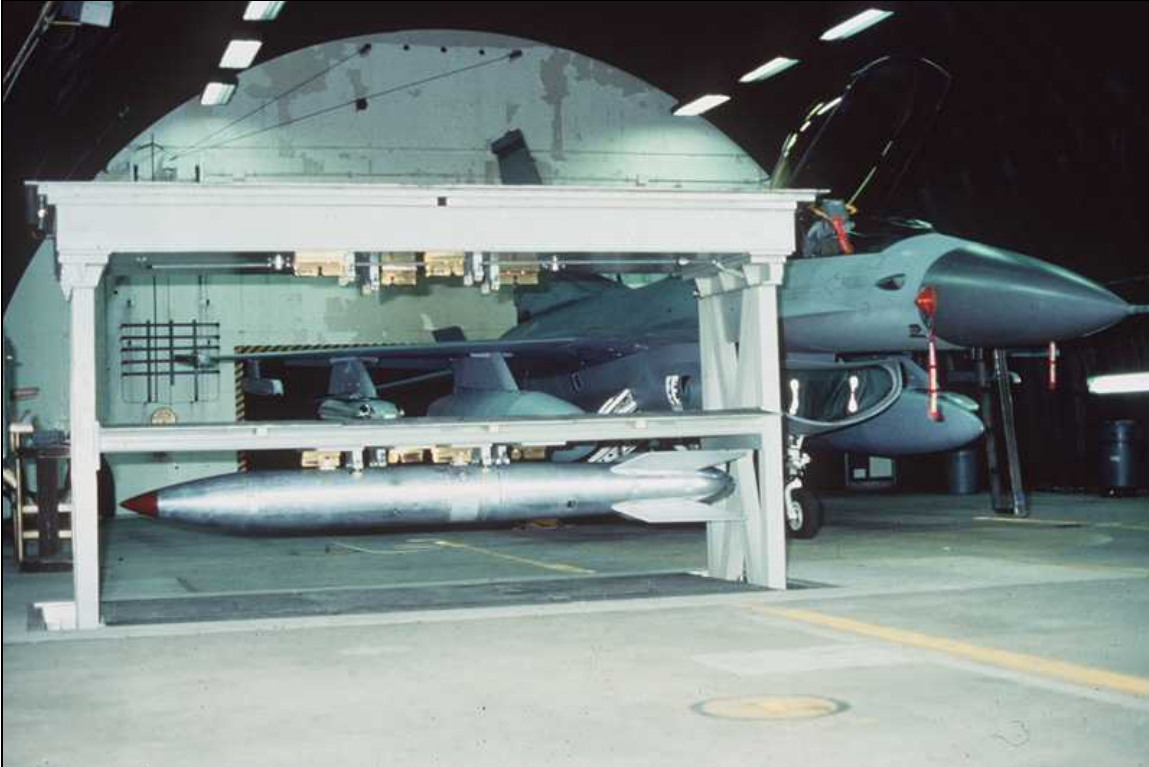
Figure 3: Elevated Weapon Storage Vault in Hangar
