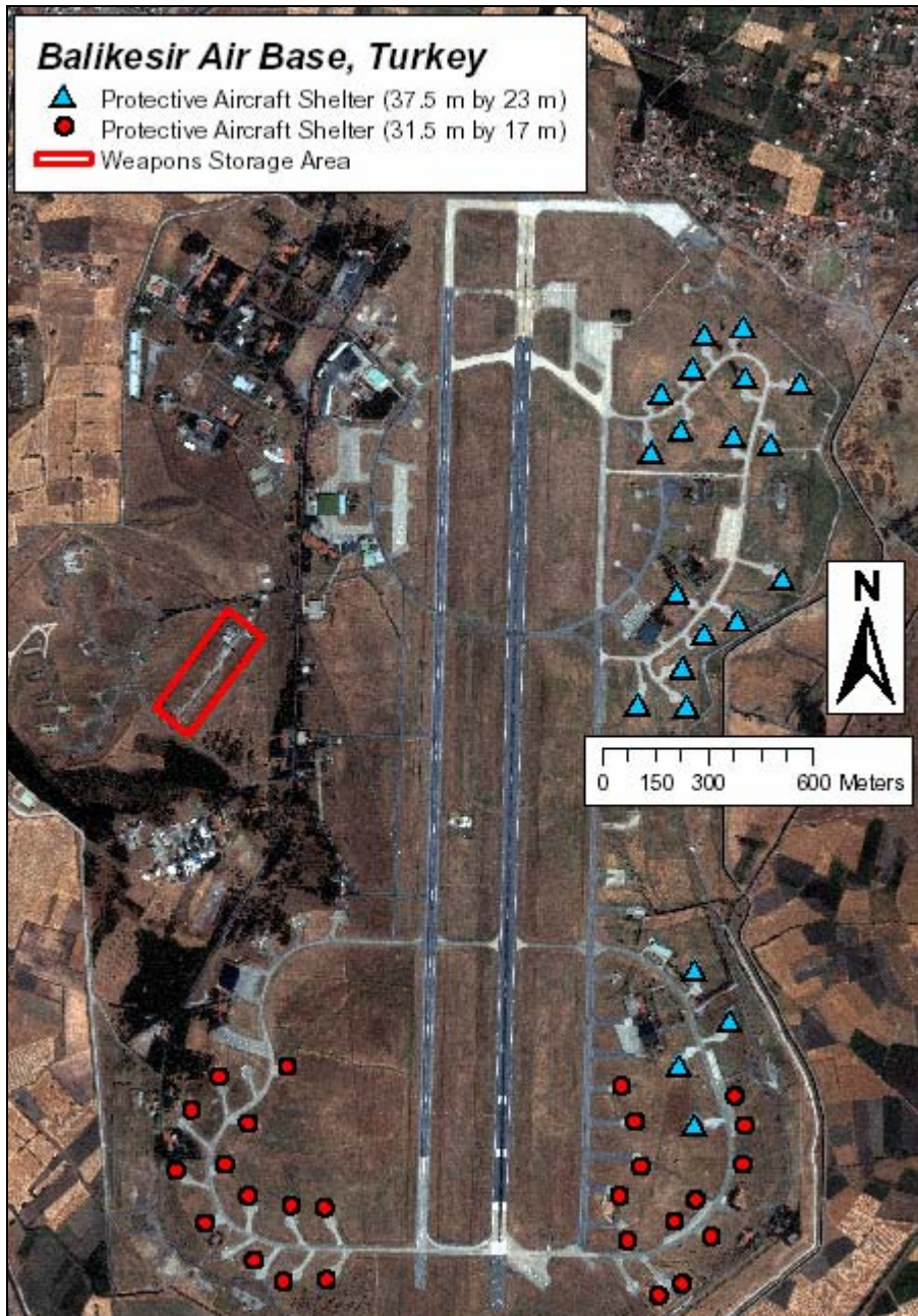
Balıkesir Air Base, Turkey (July 17, 2000): This base is located in western Turkey (39°37'N, 27°56'E). There are 47 Protective Aircraft Shelters (PAS) on the base, 21 of which are large (37.5x23 meters) and 26 smaller (31.5x17 meters) shelters. Six of the shelters are equipped with WS3 Vaults for nuclear weapons storage (maximum capacity of 24). The vaults were completed in 1997. Prior to that, nuclear weapons were stored in the Weapons Storage Area. The base stored 20 B61 nuclear bombs until 1995 for delivery by Turkish F-104G Starfighters (later F-16C/D) of the 9 th Wing. Today, weapons are stored at Incirlik Air Base but still earmarked for delivery by the 191 st and 192 nd squadrons of the 9 th Wing. Source: Space Imaging.
